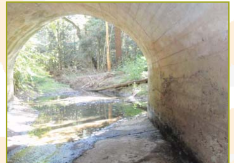
The Tunnel Drain showcasing the water level of the recent floods.
